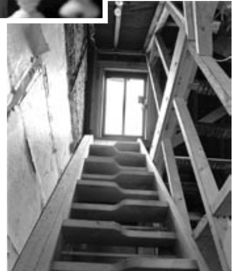
RIGHT: A view to the roof from the Scholarship Centre.
